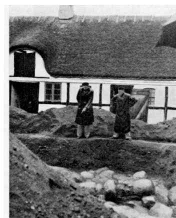
Fig. 14. — Unearthed foundation stones of the church tower. The building in the background includes the cowshed, the dairy and the privy — as adjacent sections.
