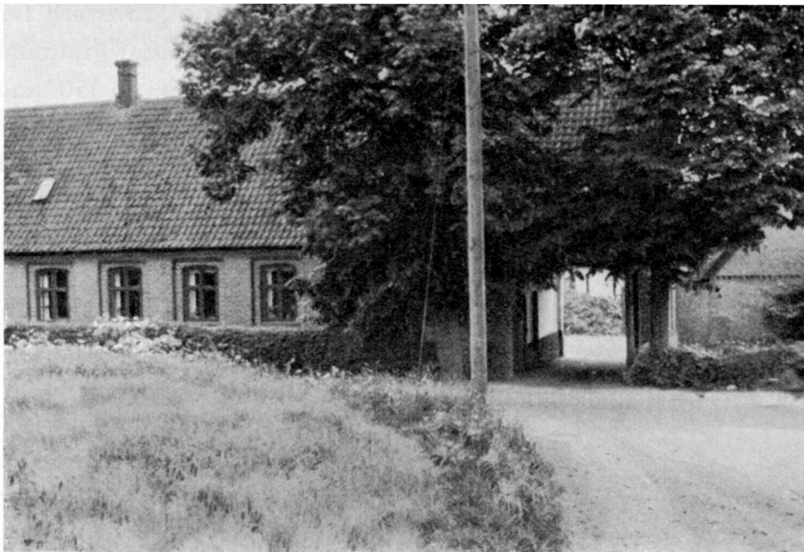
Fig. 5. — The only entrance to the farmyard. Here the choir of the old church was excavated.
